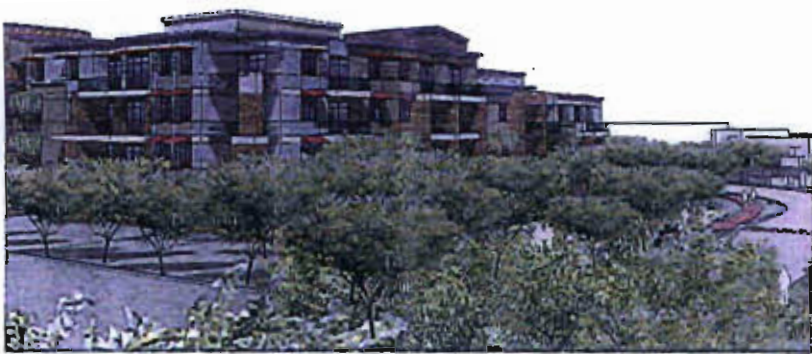
View Looking East on Rose Lane
