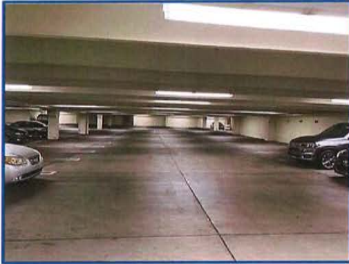
Brown Street Garage
