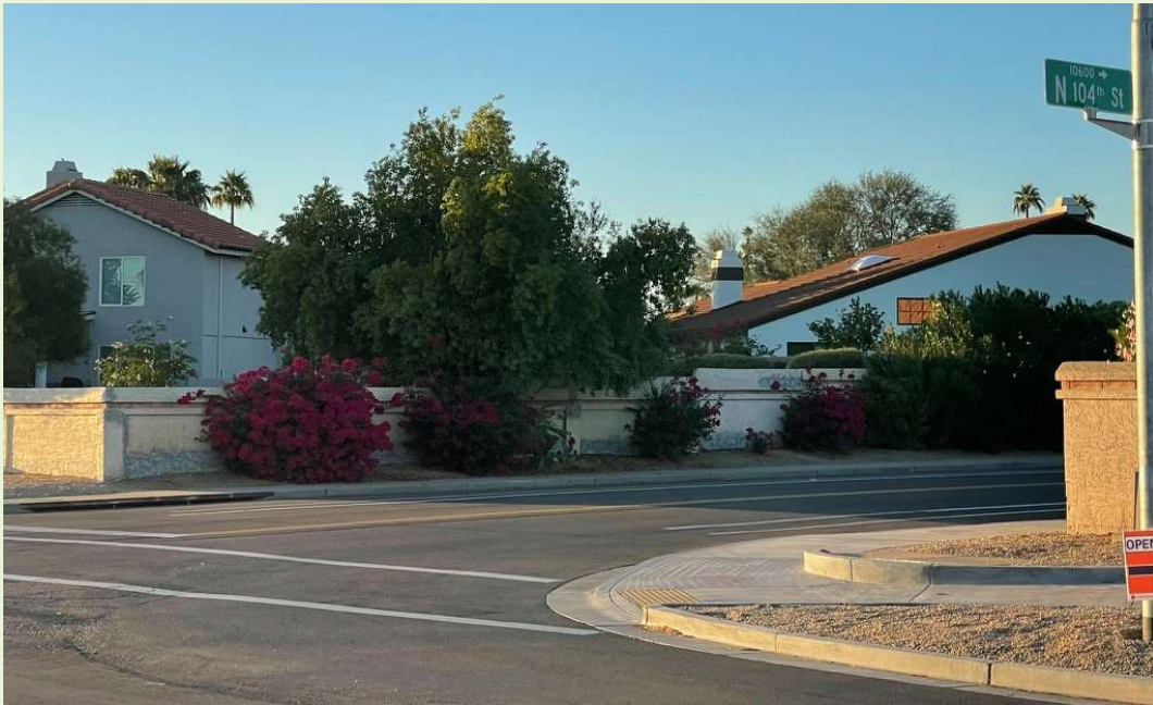
N 104 th St wall visible from all lanes of westbound Shea Blvd
