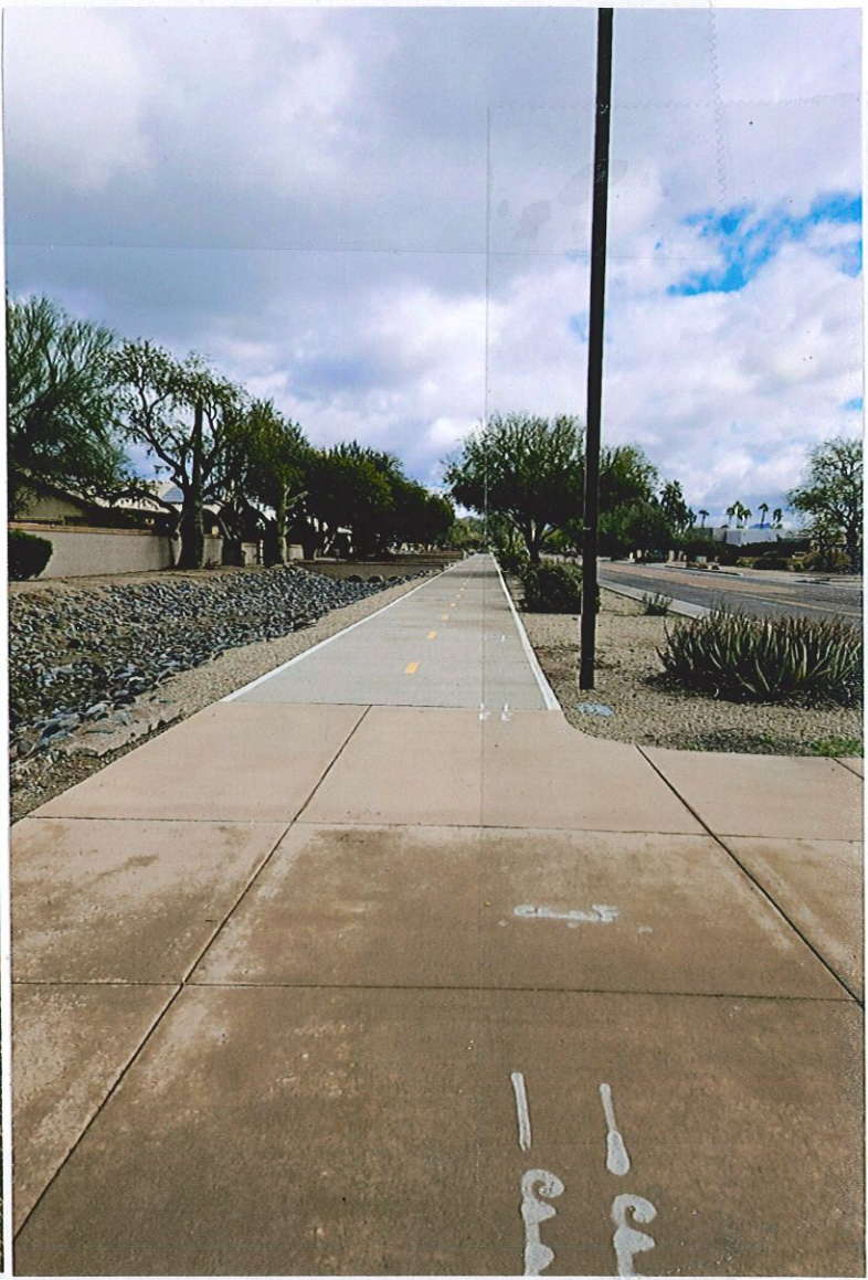
SIDEWALK ON NORTH SIDE OF CACTUS ROAD – 100% FREE OF GARBAGE AND PARKED VEHICLES
