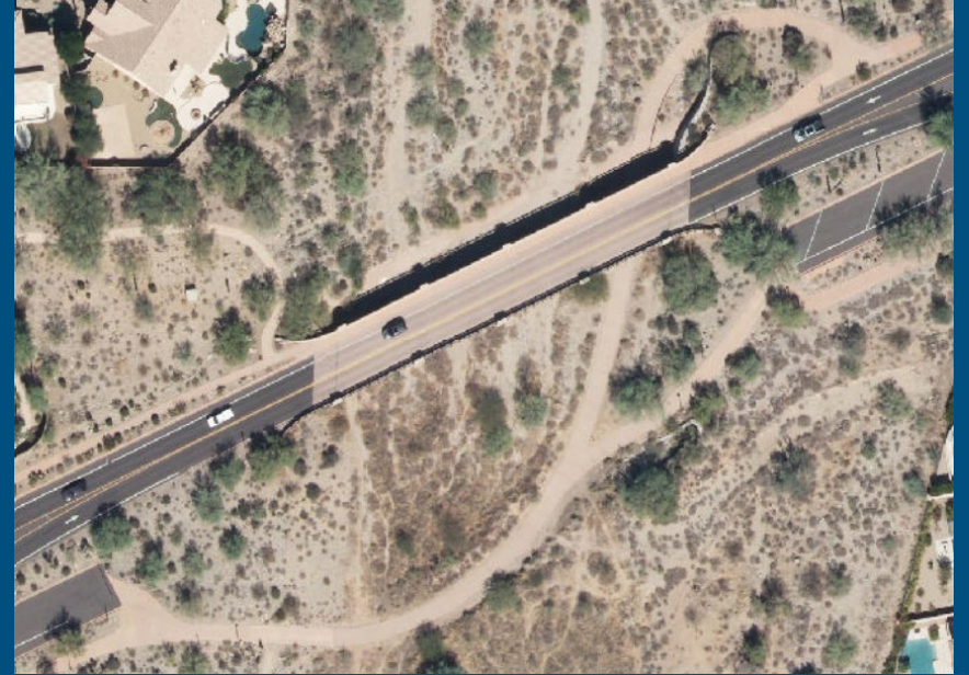
Legacy Blvd Bridge over Reata Pass Wash
