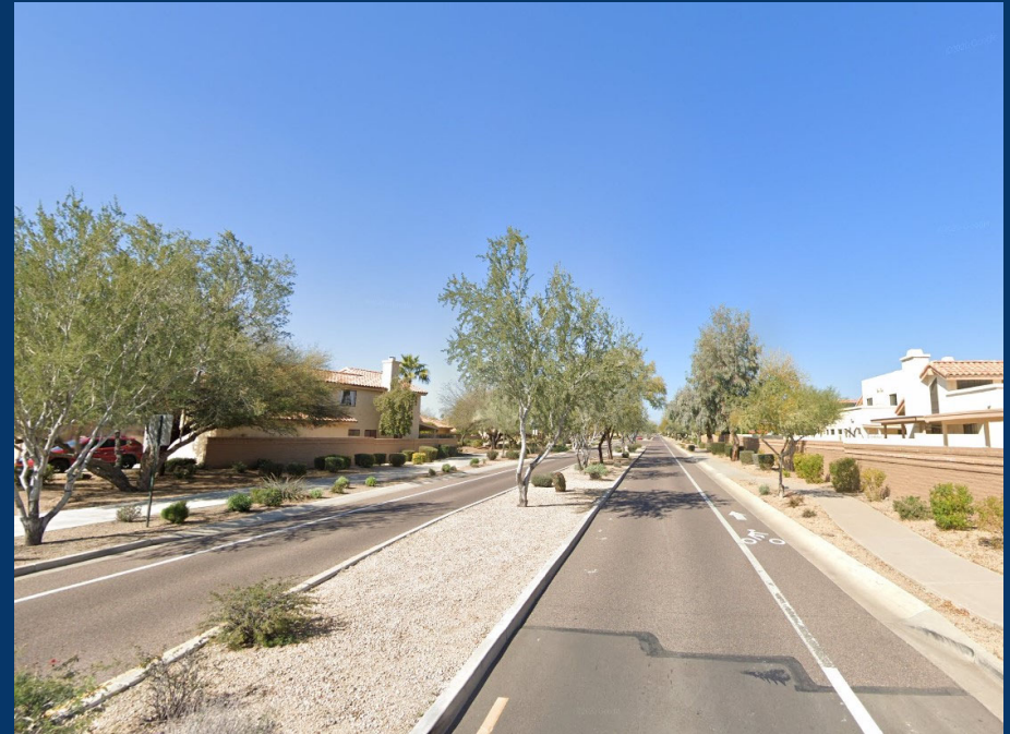
Minor Collector 96 th Street - After
