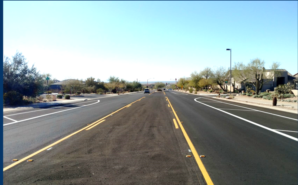
Minor Collector 124 th Street - After
