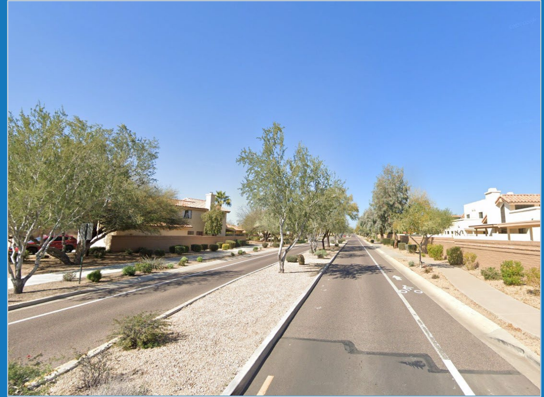
Minor Collector 96 th Street - After
