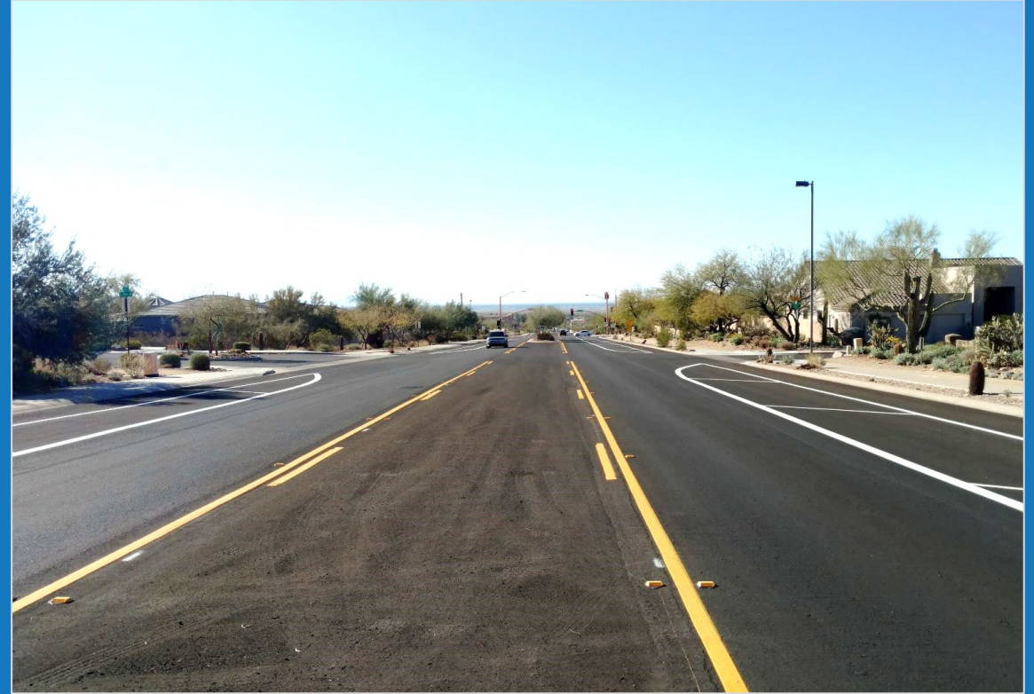
Minor Collector 124 th Street - After
