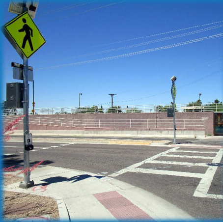
Rectangular Rapid Flashing Beacon
