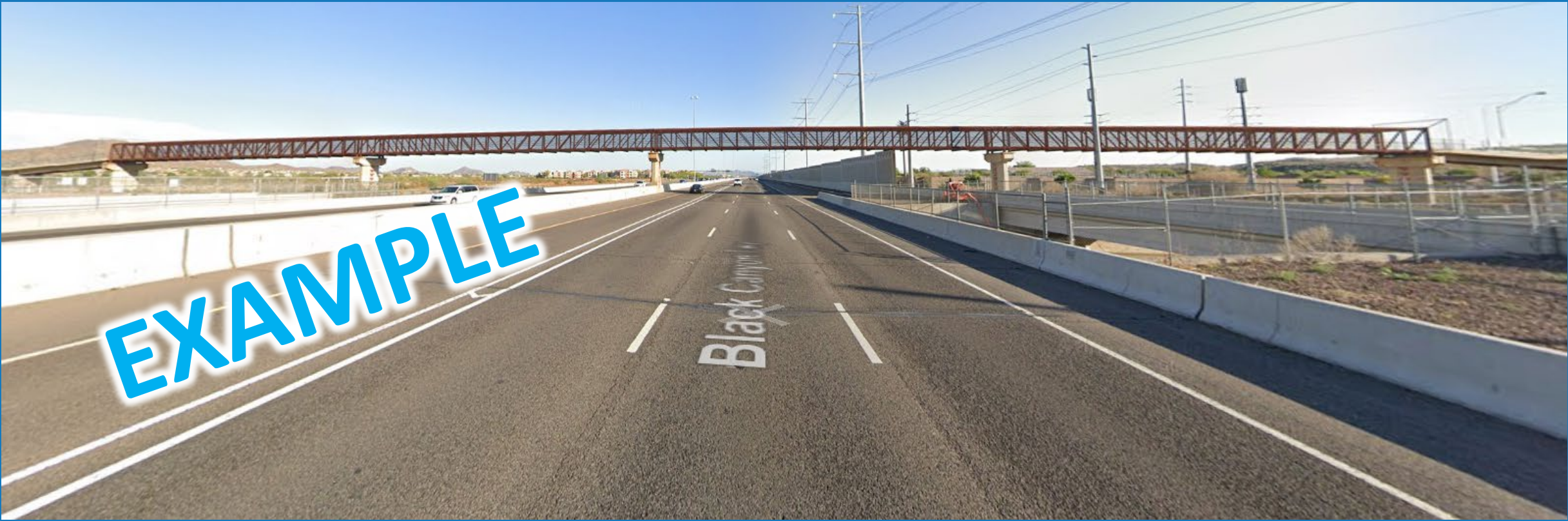
Fly Over Bridge: I-17 North of Jomax Road – 900’ Expanse
