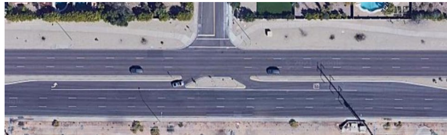
Aerial view of Shea Blvd and 104 th Street – LLO Site
