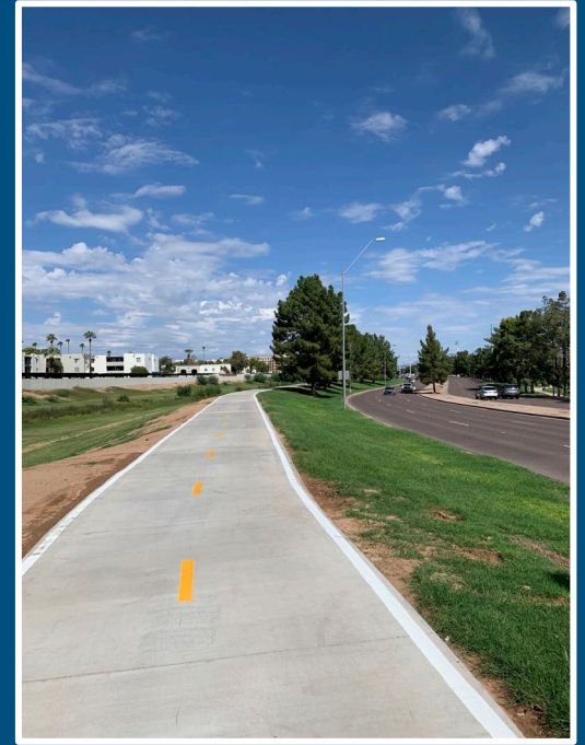
Camelback to Glenrosa After – completed September 2022
