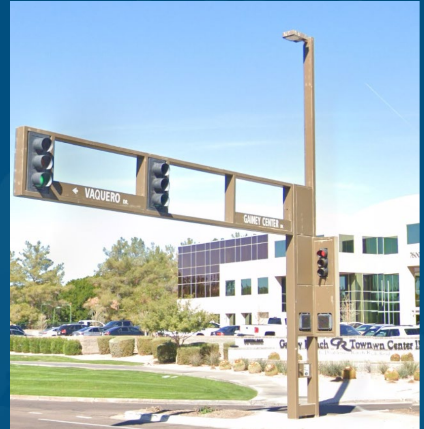
Double Tree Ranch Rd Intersection
