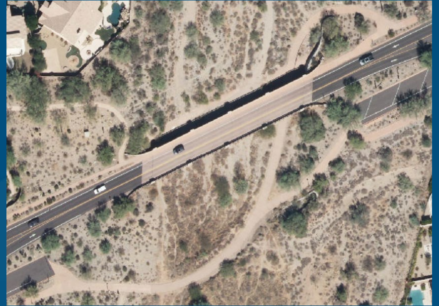
Legacy Blvd Bridge over Reata Pass Wash
