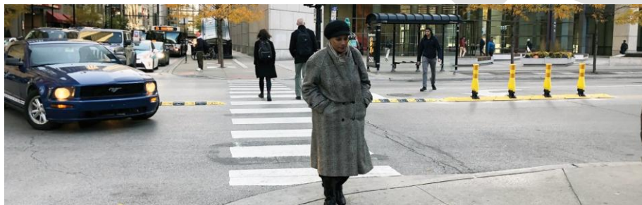
Figure 10 – Centerline hardening in Chicago, IL Credit: Chicago Department of Transportation
