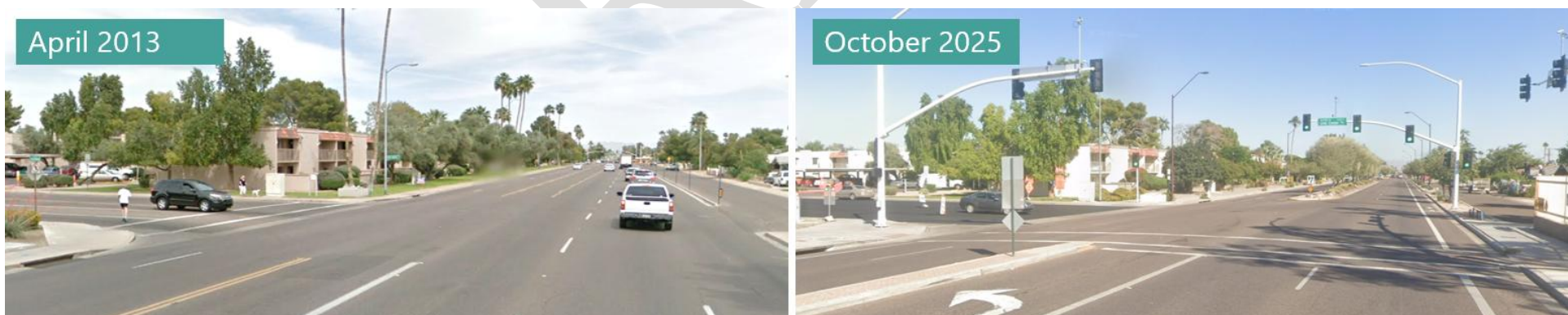
Figure 11 - Access Management & Intersection Improvements on Thomas Rd. (Courtesy of Google Street View)
