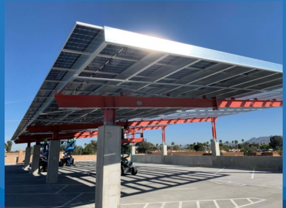
View of shade structure
