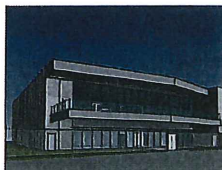
View from Apron
