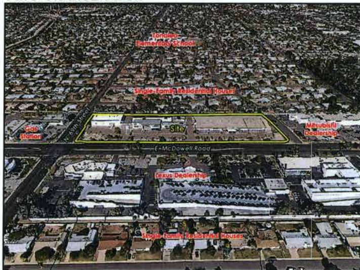
OBLIQUE DETAIL AERIAL
