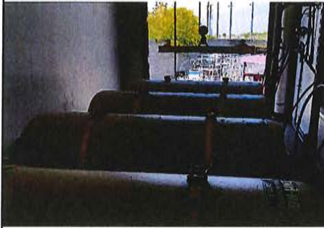
Above: Old gaseous chlorine tanks
