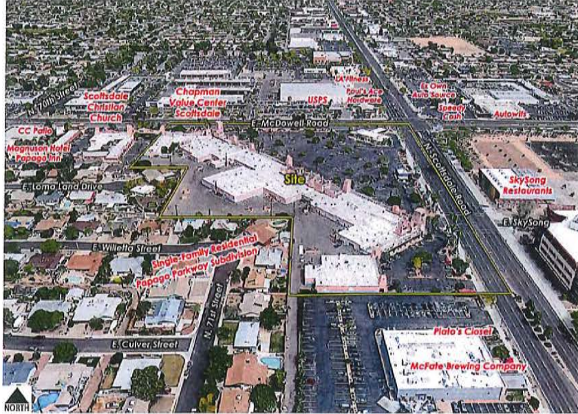
Detail Aerial (facing north)
