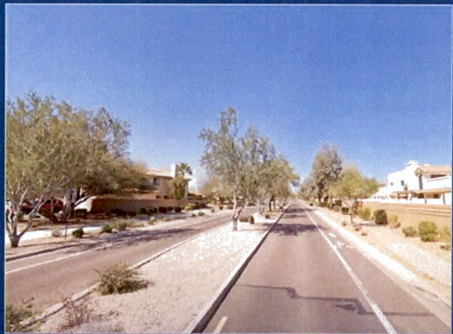
Minor Collector 96 th Street - After
