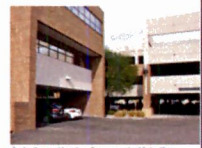
A single parking bay incorporated into the building design, and internal to the site, beneath the second floor.
