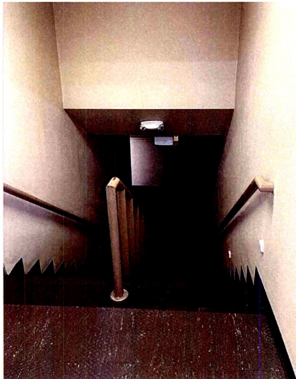
Existing FS 606 stairs down to bunks
