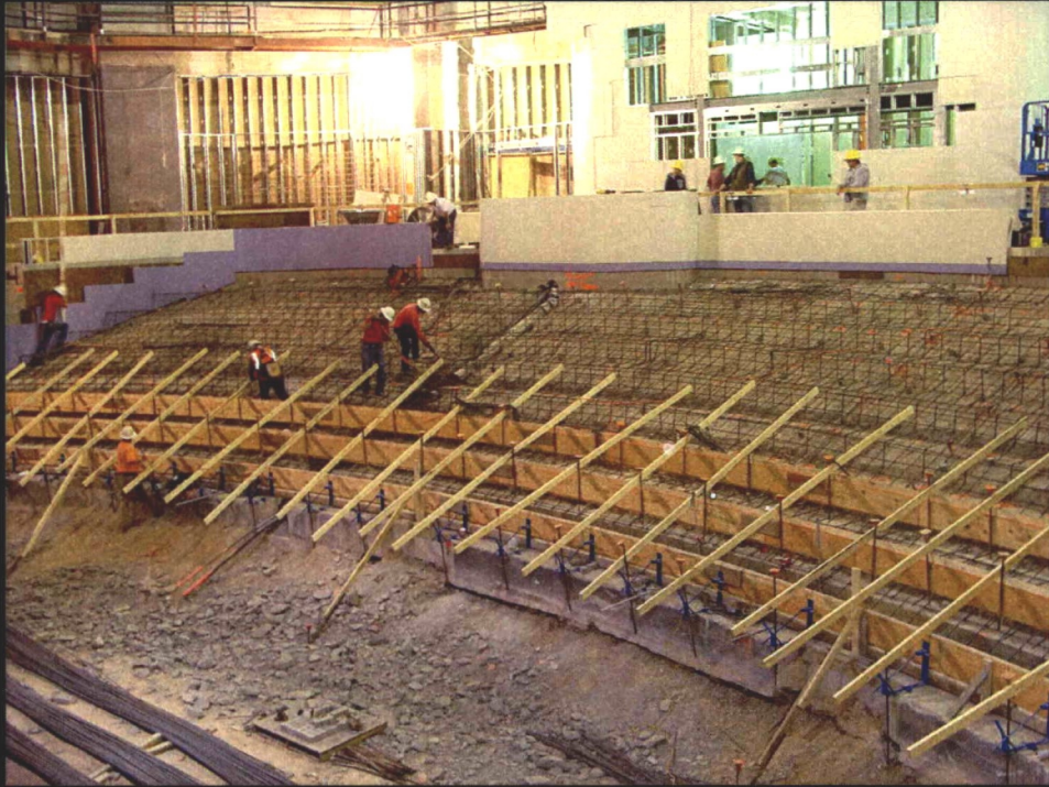
Main Theater Renovations
