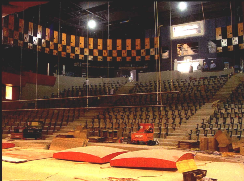
Main Theater Renovations
