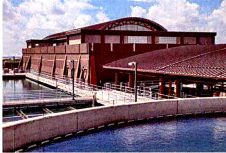
2011 CAP Water Treatment Plant Expansion
