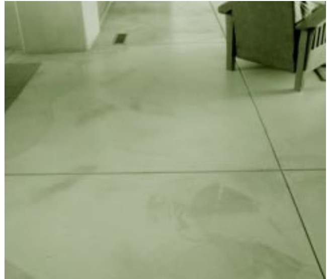
Finished concrete floors create smooth surfaces that are easy to maintain and stay cooler in the summer months.
