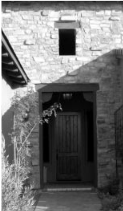
By incorporating recessed doors and windows into the design of your home, you can minimize solar heat gain.
