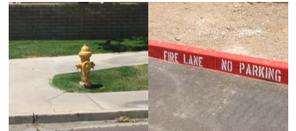
Unobstructed Fire Hydrant
