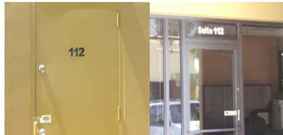
Suite numbers should be clearly marked on both front and rear doors.
