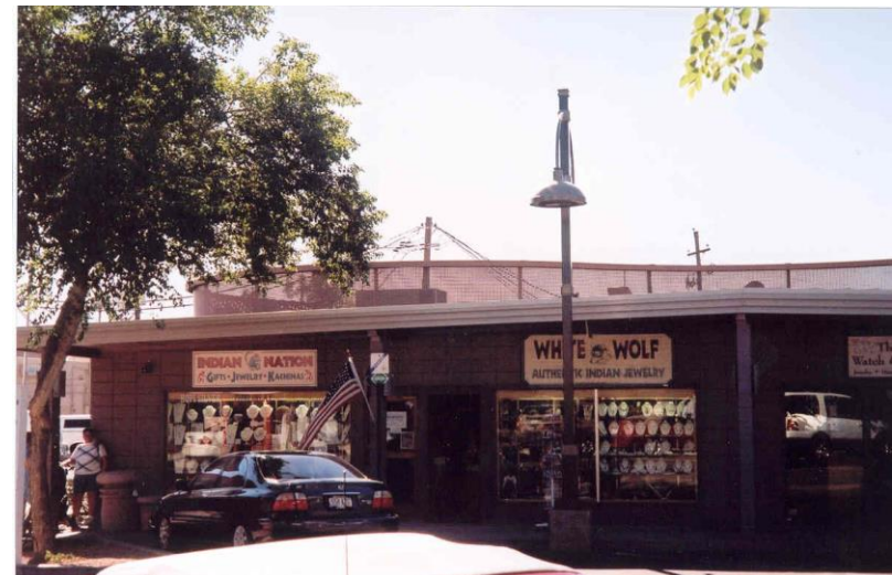
Fifth Avenue (north) elevation of building 3
