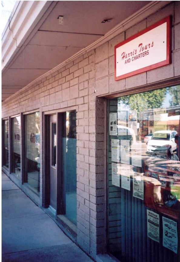
West elevation of building 3
