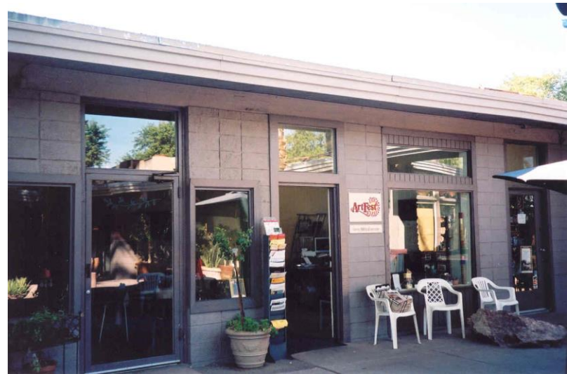
North side of building 6 facing courtyard; varied openings
