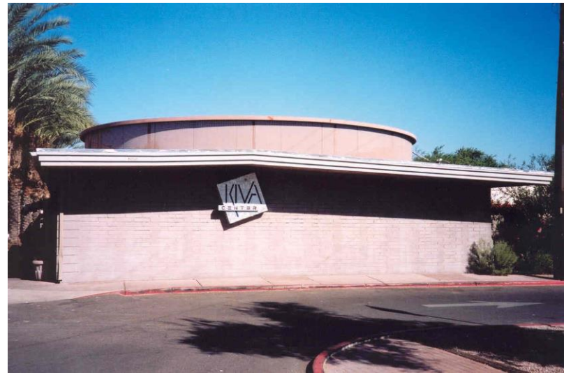
Rear (south) elevation of building 4; entry to courtyard on left
