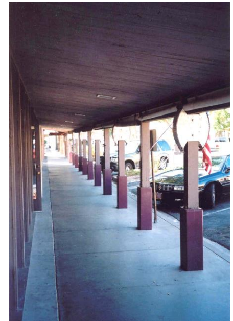
Colonnade along Craftsman Court for building 7
