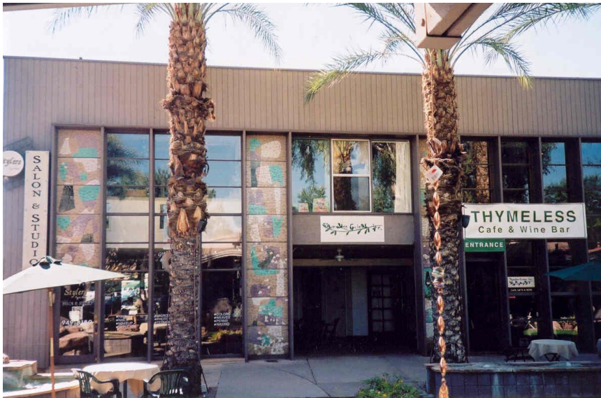
North elevation of building 5 facing courtyard
