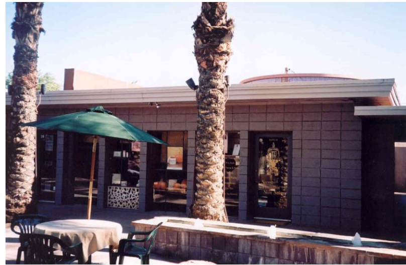
West elevation of building 3
