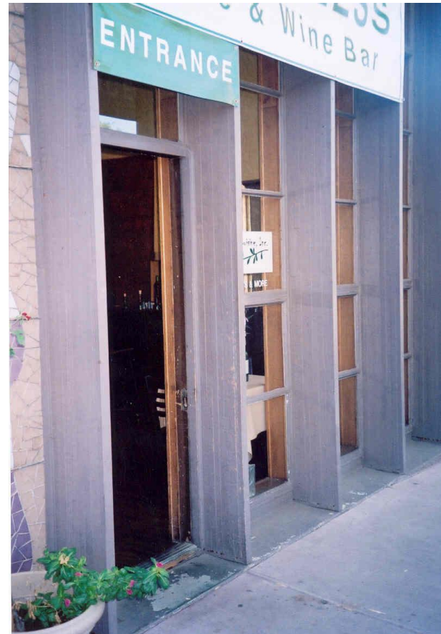
Projecting laminated wood frame on window wall and steel sash windows
