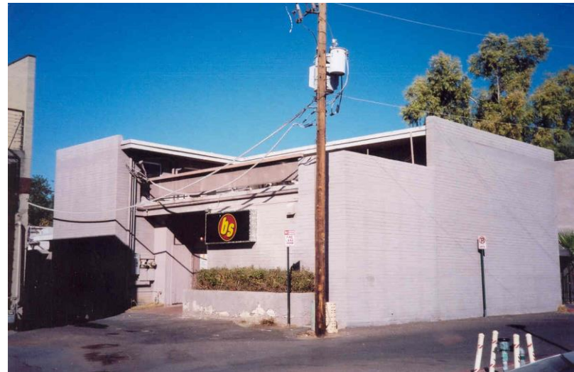
South and east elevations of building 5a
