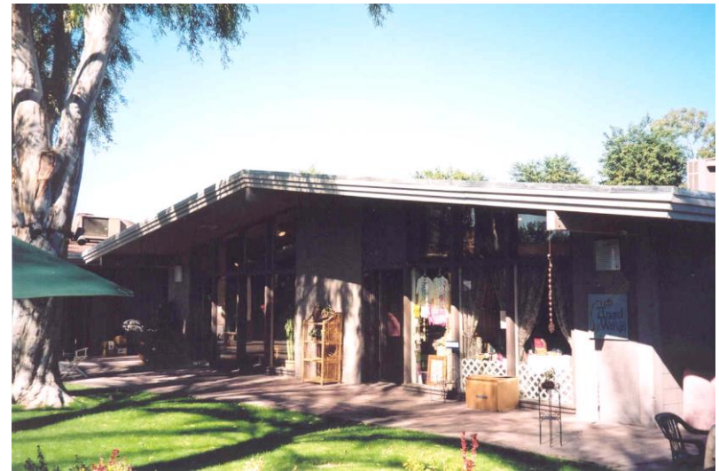
Rear (south elevation) of building 2
