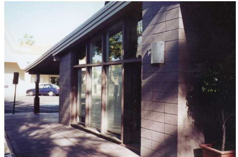
Stacked masonry bond and window wall on south elevation of building 1
