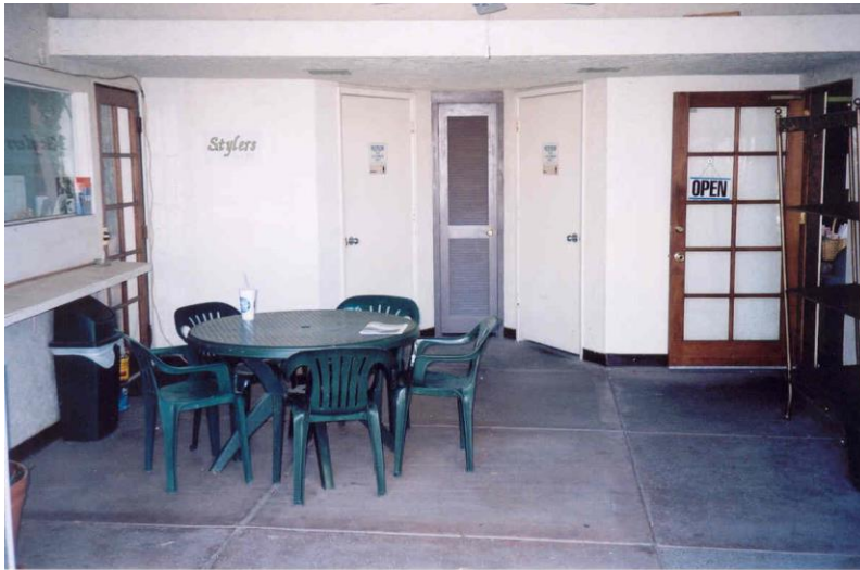
Recessed first floor courtyard on north elevation
