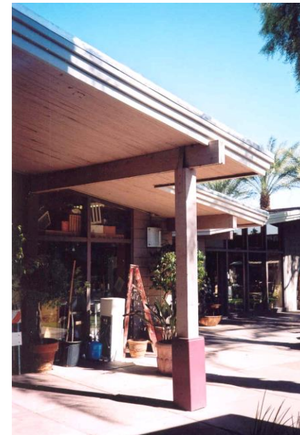
South entrance to building 1
