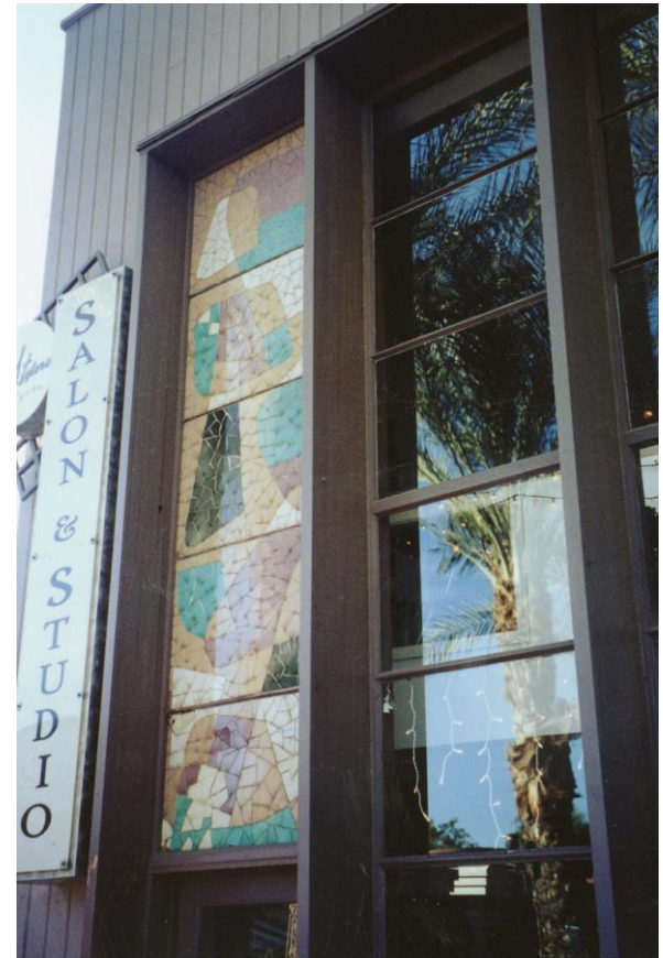
Detail of mosaic tile panel on east end of north facade
