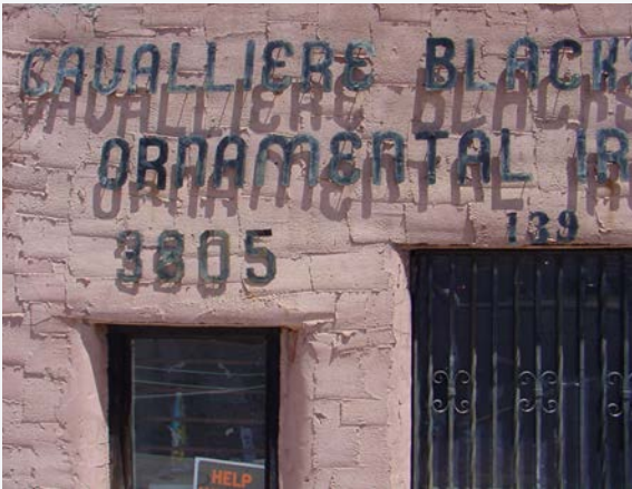
This sign features hand-crafted, torch cut letters, mounted above a stucco finished adobe wall - an appropriate sign for an historic blacksmith shop.
