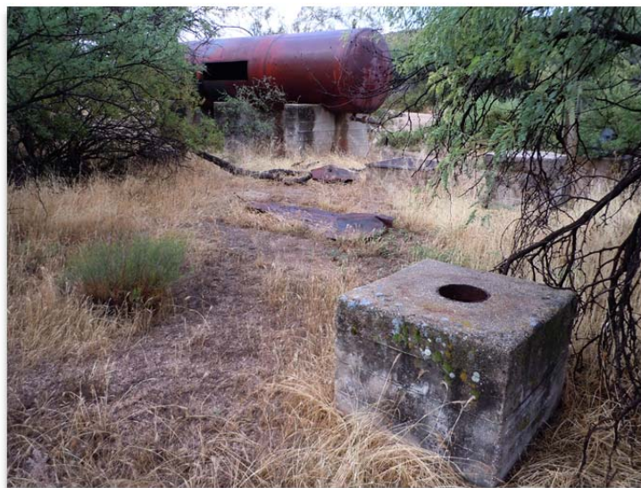
FIGURE 16. HISTORIC WATER COMPLEX AT BROWN'S RANCH
