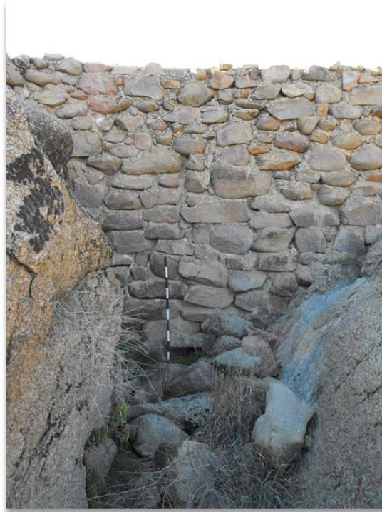
FIGURE 12. HISTORIC ROCK WALL
