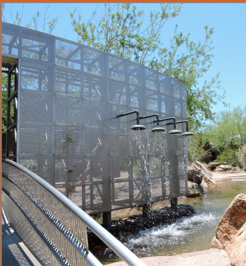
The CAP Water Treatment Plants are located at the Scottsdale Water Campus in north Scottsdale.
